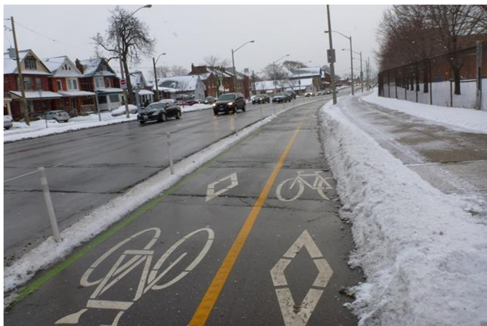
Figure 4-18: On-road separated bike lane maintained year-round in Hamilton, Ontario. Source: IBI Group
