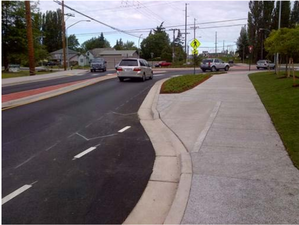
Figure 4-44: Example of bicycle ramp at roundabout facility Source: Custom Concrete
